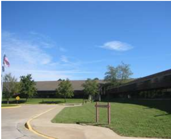
Roberts State Office Building - DMH
