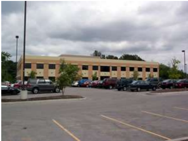
Jennings State Office Building
