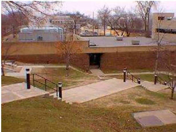
Environmental Control Center (ECC)
